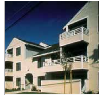
31 units per acre Paula Ave. Apartments San Jose, CA
